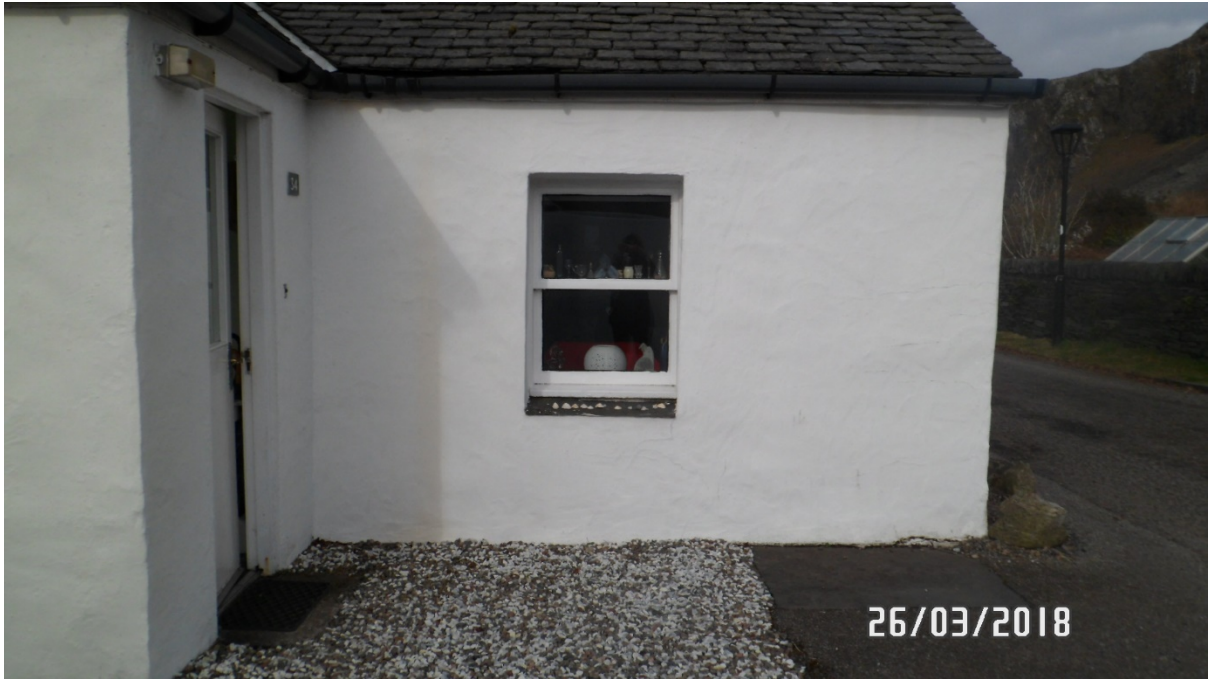
Close up of white timber sliding sash and case unit to front elevation
