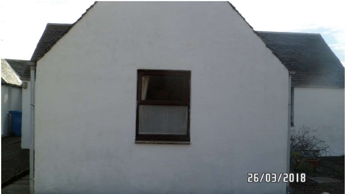
Close up of brown painted timber top hung window to front elevation
