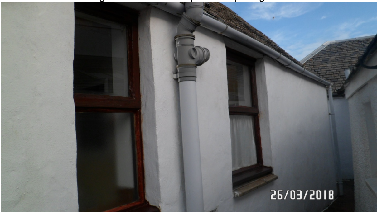
Close up of windows to rear elevation showing brown timber painted top hung windows
