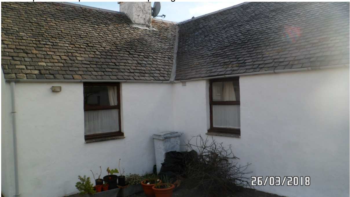
Side elevation showing 2 no. brown painted timber top hung windows
