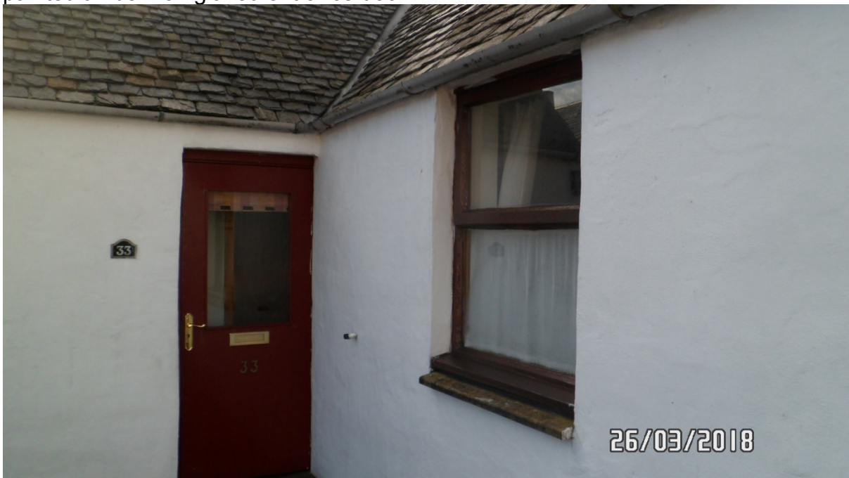
Close up of front elevation showing brown painted timber entrance door and brown painted timber top hung window
