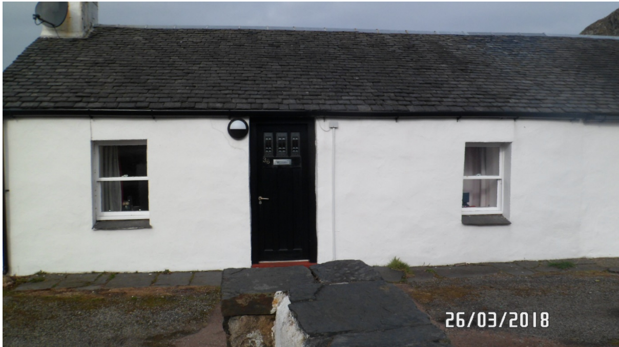
Front elevation showing 2 no. white painted timber sliding sash and case windows and 1 no. black painted timber door with small glazed panels.
