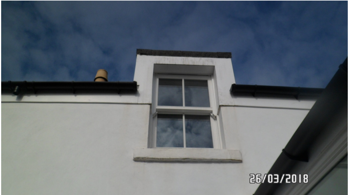
Close up of first floor white timber sliding sash and case window to left of entrance porch
