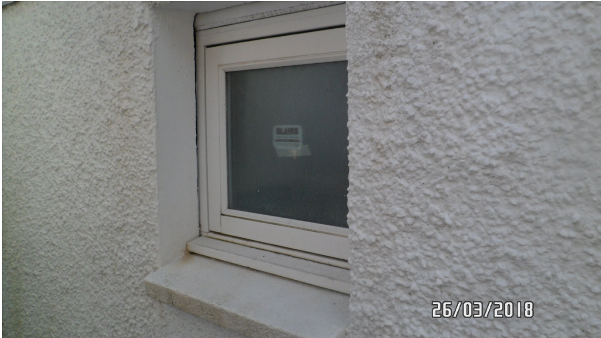
Close up of window to obscure glazed white timber window to rear elevation of single storey projection
