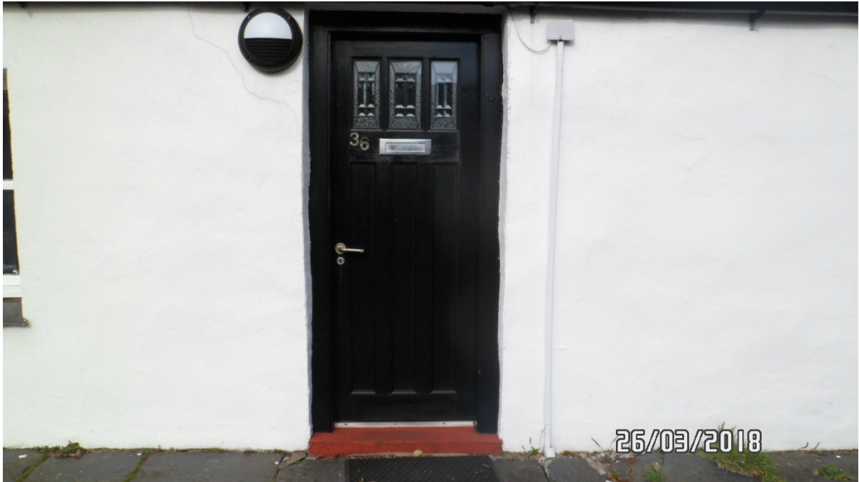
Close up of black painted timber entrance door to front elevation
