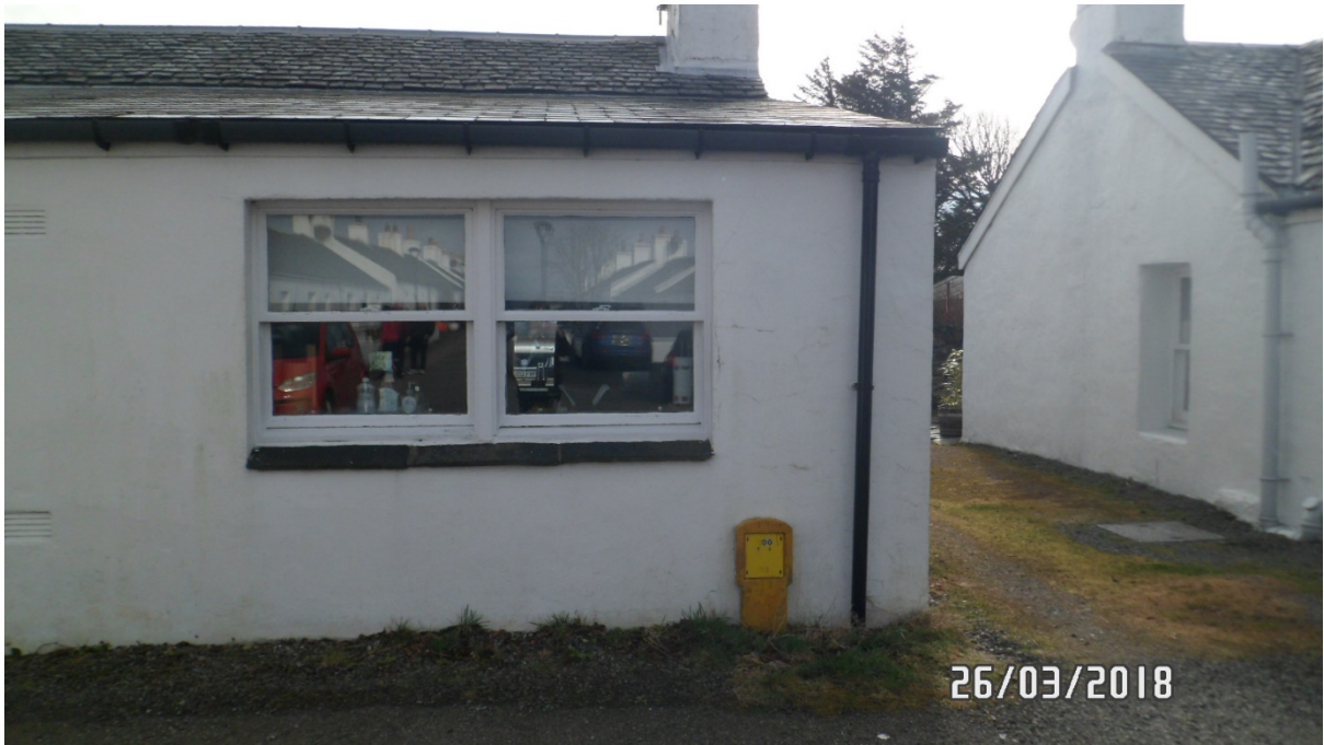
Close up of double white painted timber sliding sash and case window to rear elevation
