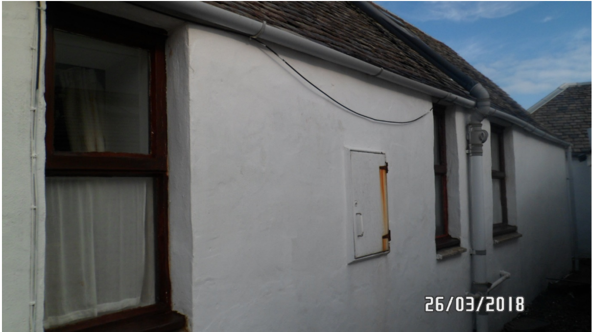
Rear elevation showing 3 no brown timber painted top hung windows
